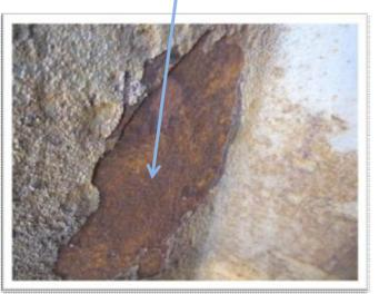
Hopper side paint and scale must be removed where edges are lifting and can be removed with a paint scraper.
