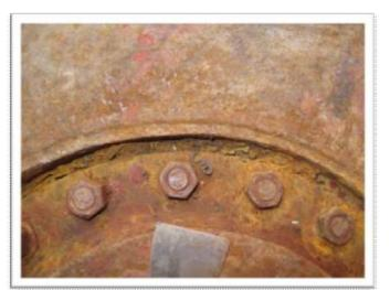
Manholes should be checked for rust and debris in the grooves.
