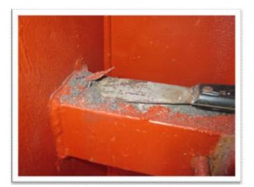
Paint scraper can get under loose paint / rust. In this case there is grit from blasting painted over.
