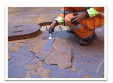
Tanktop sheet rust must be removed. In some cases a hammer or chipping machine may be required to ensure all loose rust is removed.
