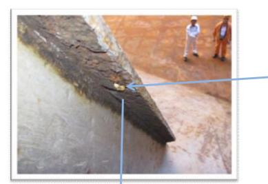
Always check behind frames for loose scale and also previous residues which may be lodged behind the rust scale.
