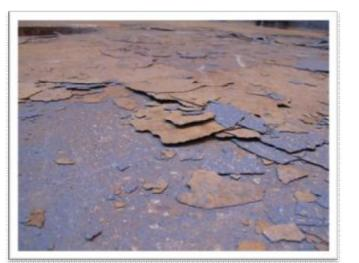
Tanktop sheet rust is best removed dry with chipping hammers and scrapers.
