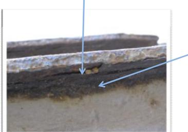
Some sheet rust behind frames may also extend to the angle section of the frame
