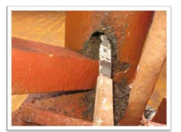
Rusted out structures like spiral ladder posts must be cleaned out carefully and repaired.
