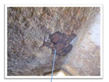
Bulkhead blisters that sound hollow should be chipped back. These are easy to identify by tapping with a paint scraper or chipping hammer.
